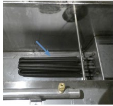
Fig 3.3 Heating element
